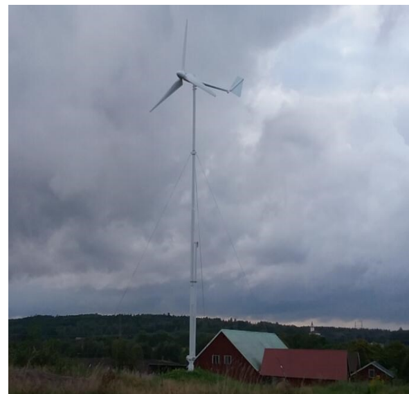
Fig. 7. The WT with a nominal output of 2 kW - an example of the appearance after installation [25]. (Source: https://www.windpowercn.com/products/21.html )
